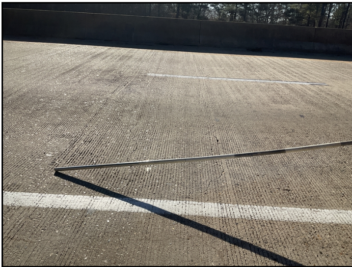
Span 4 deck large transverse cracks.
