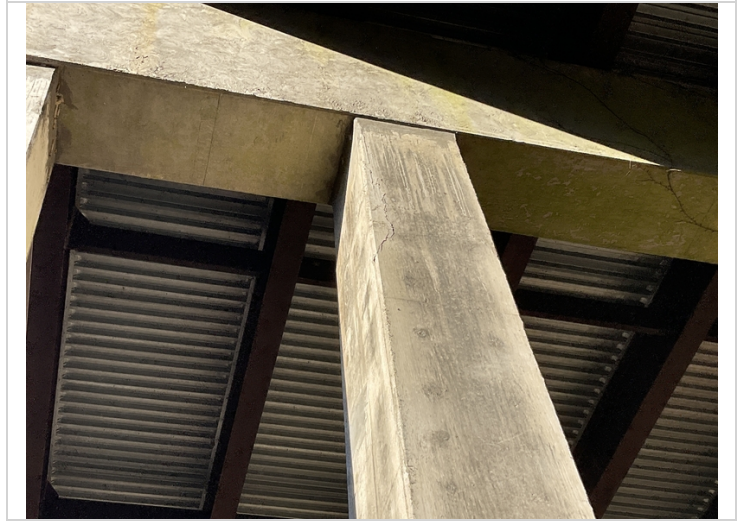
Bent 2 column 3 delam on ahead side.
