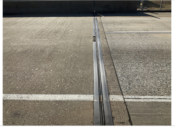
Bent 1 joint armor has two foot of armor missing.
