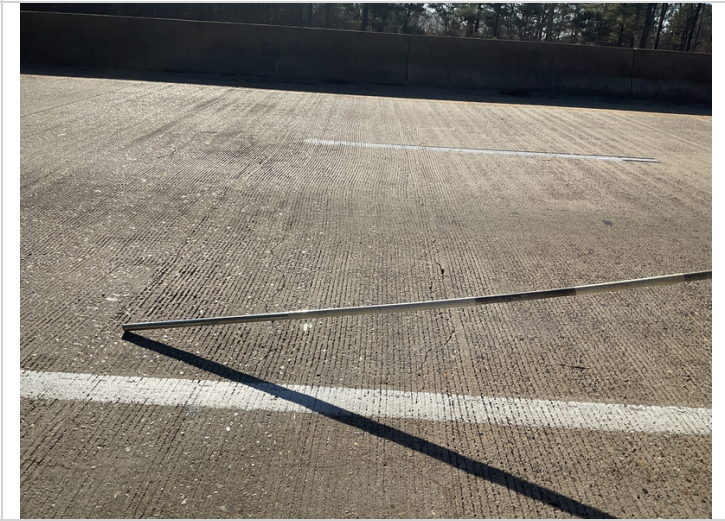
Span 4 deck large transverse cracks.
