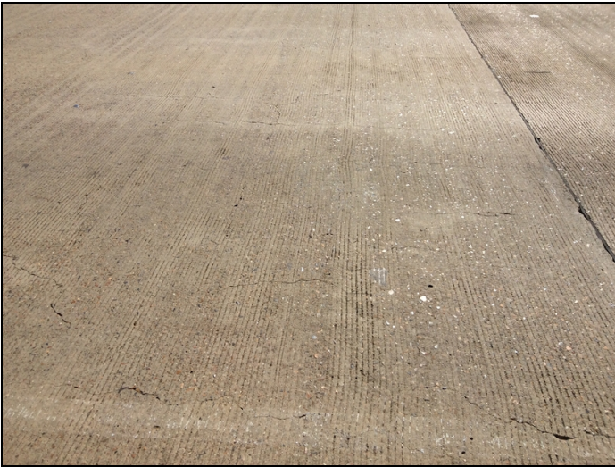
Span 3 longitudinal and transverse cracks up to 0.050"
