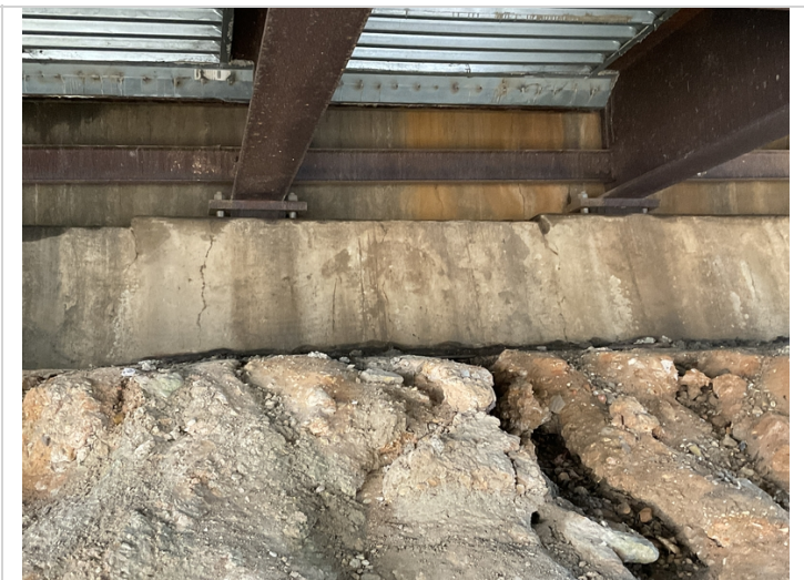
Small vertical cracks in abutment at bent 5.
