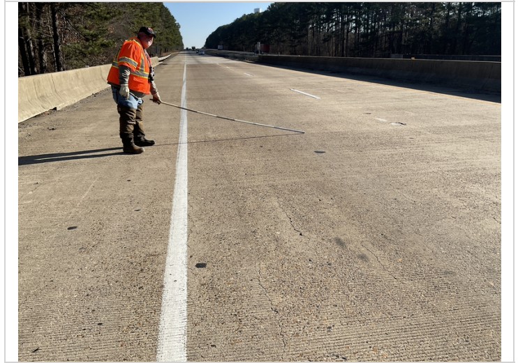
Span 2 large longitudinal and transverse cracks.
