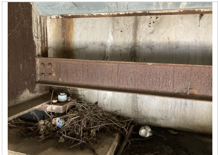
Cracks with efflorescence in back wall at bent 1.
