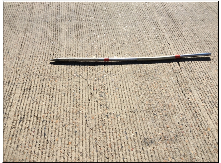
Span 3 longitudinal and transverse cracks up to 0.050"
