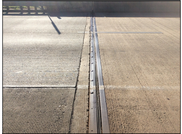
The joint armor is loose at bent 5.
