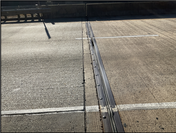
Joint armor at bent 5 loose under traffic.
