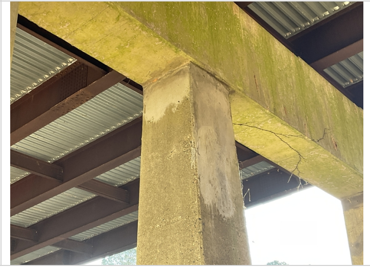
Bent 2 column 2 delam on back side.
