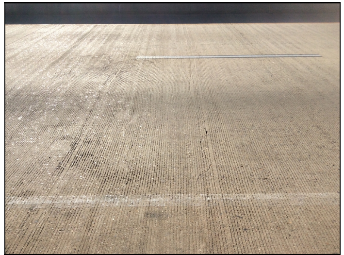
Transverse cracks in span 3.
