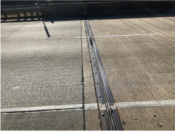
Joint armor at bent 5 loose under traffic.
